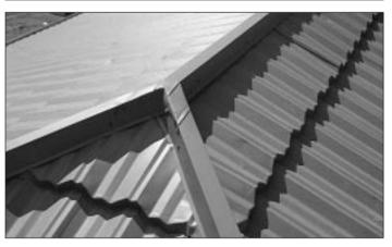
Then cut ridge cap to fit over hip trims. Install then lay the rest of the ridge caps.
