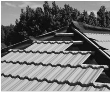
As each length of underlay is laid, replace the battens on the top of the building paper against the marking nails.
