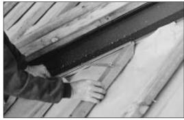
After laying valley tiles gently tap a piece of wood onto the edge to ensure a perfectly even downturn.
